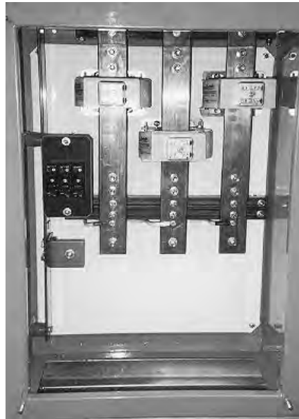
Figure 4.15: Typical CT Installation in a cubicle type switchboard
