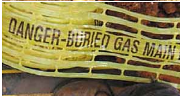
Top: Trenching and laying of new pipes and cables. Left: Non-metallic gas pipe marker. Right: Cable at incorrect depth.
