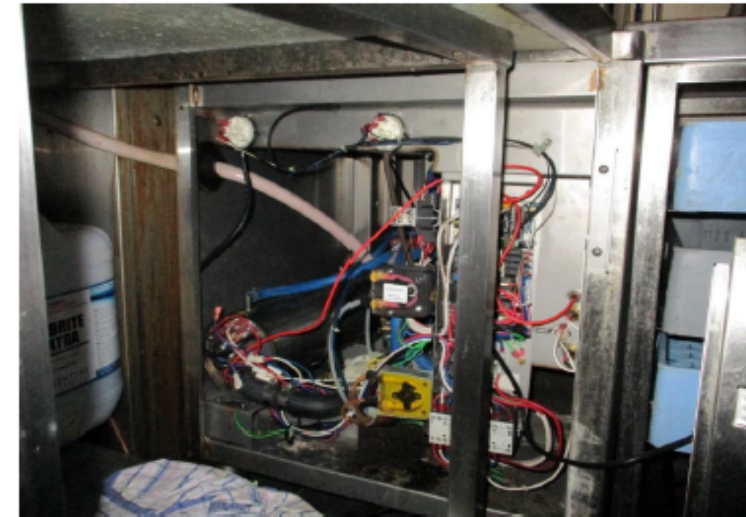
Photograph 1: The commercial dishwasher wiring and control area (3 phase supplied, covers removed)
