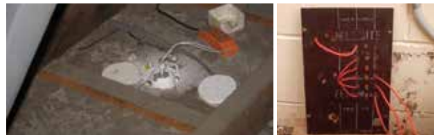
Figure 5: Asbestos millboard, asbestos resin board debris and asbestos insulation board debris in the bottom of electrical cabinets.
